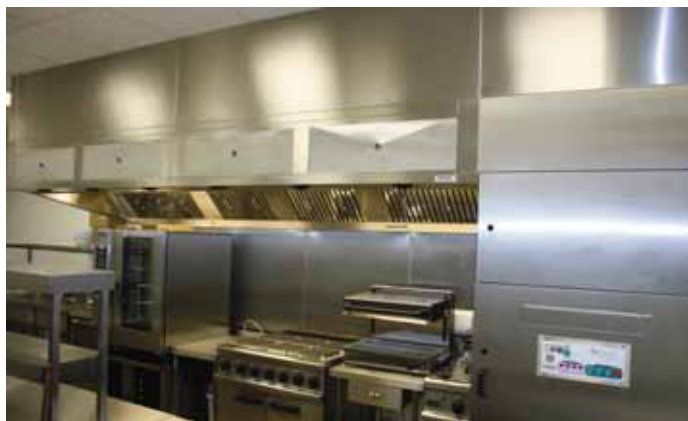
Refresh self contained kitchen ventilation system at British Medical Association in London
