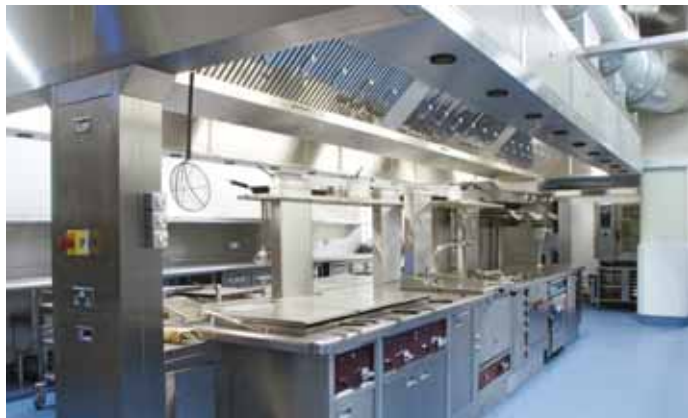
Ultrastream UV filtration system at Wadham College in Oxford
