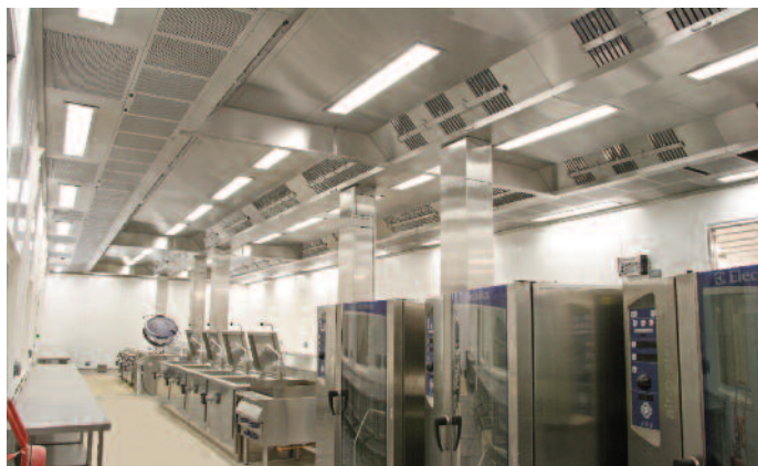
Silverline ventilated ceiling at HMP Parkhurst, Isle of Wight
