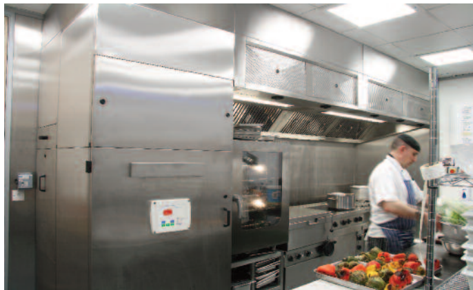
Refresh self contained kitchen ventilation system at Mills Reeve, Norwich
