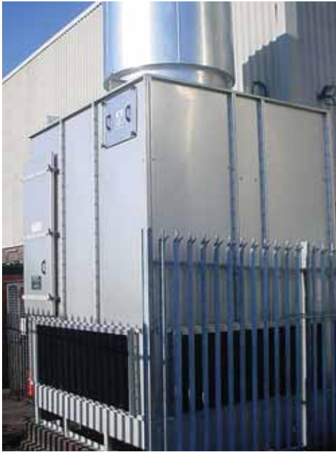
Induced draught counterflow tower, with cooling airflow being provided by top mounted directly driven axial fansets
